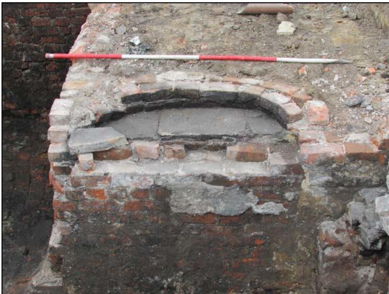
Figure 81. Curved cellar light (143) abutting wall (142). Looking north.
