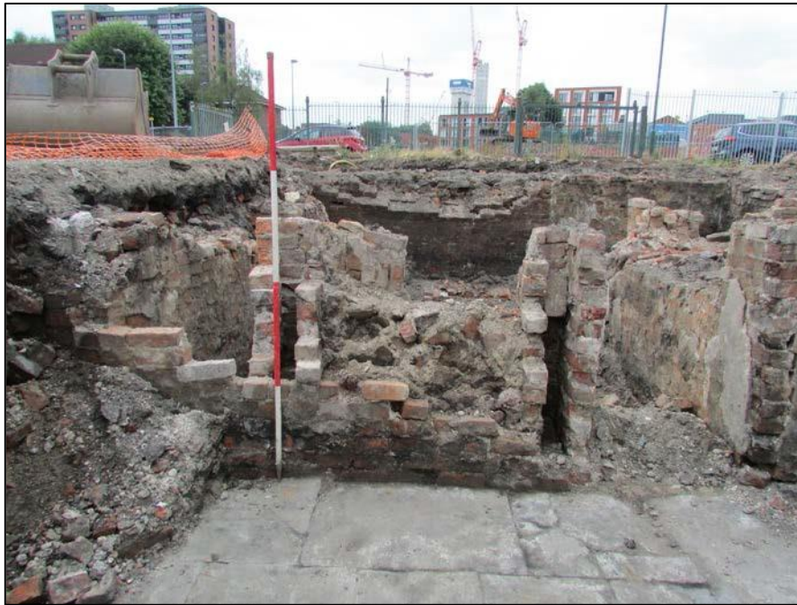
Figure 45. Rear of fireplace in House 5, visible from House 4 showing hollow uprights. Looking west.
