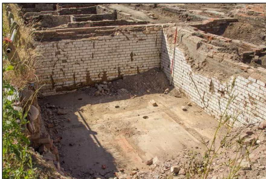
Figure 6. Bank Room 1, showing glazed brick walls, concrete floor and wall scars (010), (011) and (012). Looking southwest.
