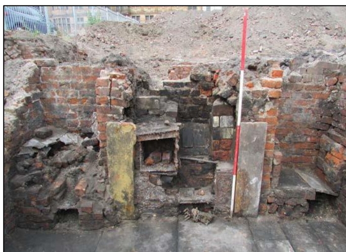
Figure 53. Detailed view of range and set pot inserted into wall (197). Looking north.
