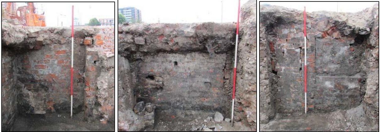
Figures 37-39. Southern, central and northern sections of wall (165) respectively, showing blocked fireplaces to either end and possible fixing holes in the centre. Looking west.
