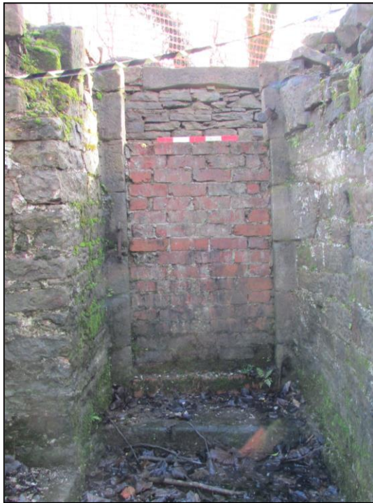
Figure 40. Blocked doorway in wall (005). Looking east.
