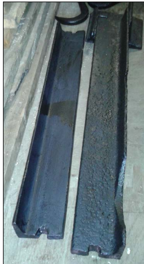
Figure 17. Examples of in situ tramway sleepers at Bugsworth Basin.
