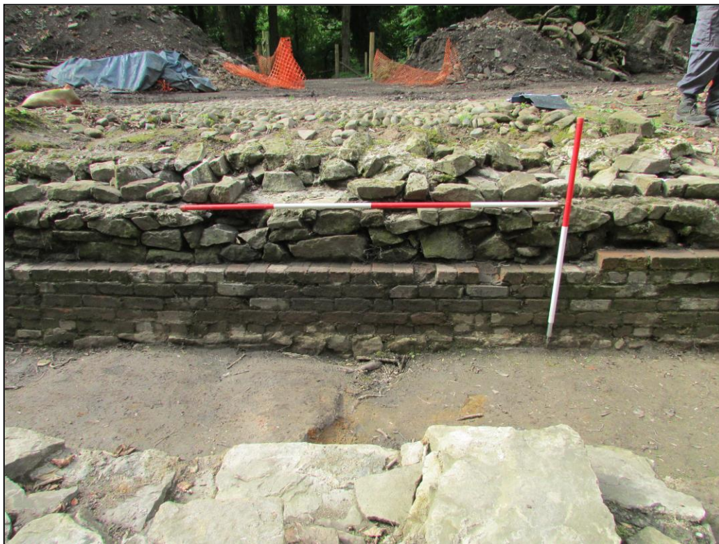
Figure 53. South-eastern face of wall (027) showing internal brick course, stone footings and rubble core with (018) in the foreground. Looking northwest.
