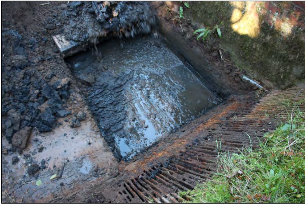
Plate 33: Concrete base directly below the silt deposit, forming the base of the weir
