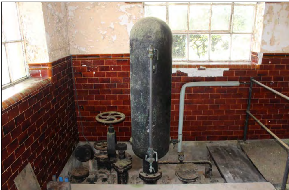
Plate 30: Outflow valve, with large air vessel
