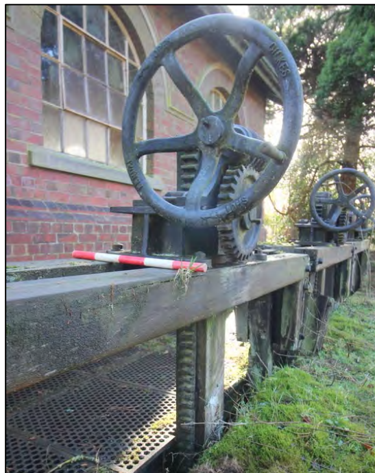
Plate 23: Detail of sluice valve
