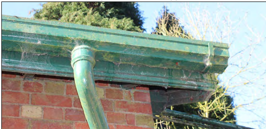
Plate 13: Detail of timber gutter and moulded eaves board
