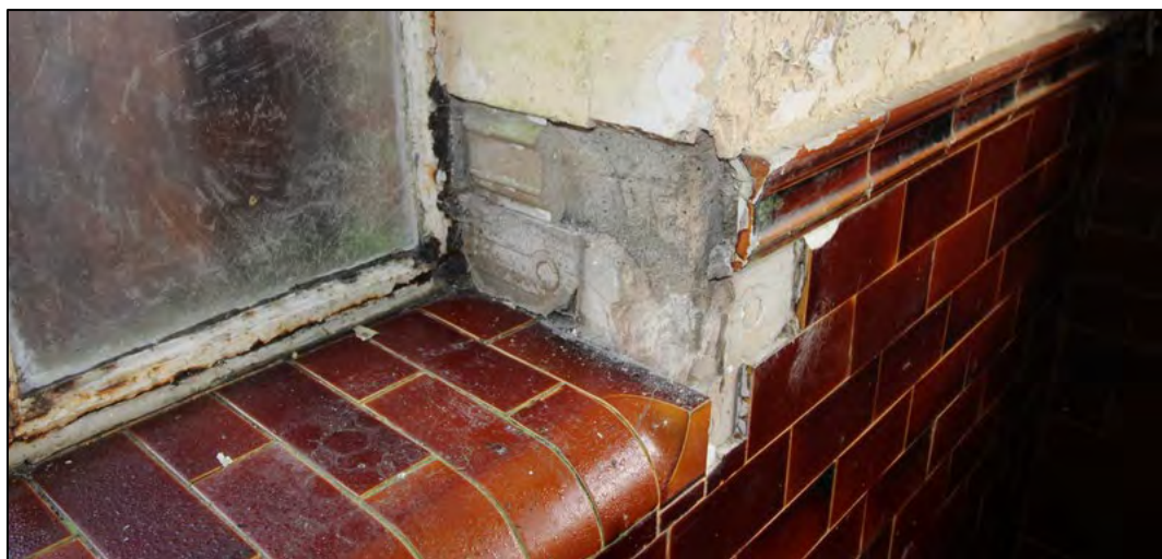
Plate 25: Missing tiles within window jamb, and partial stamp imprint in plaster
