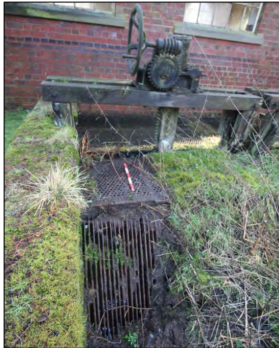
Plate 22: Iron screen and gantry to sluice gate control
