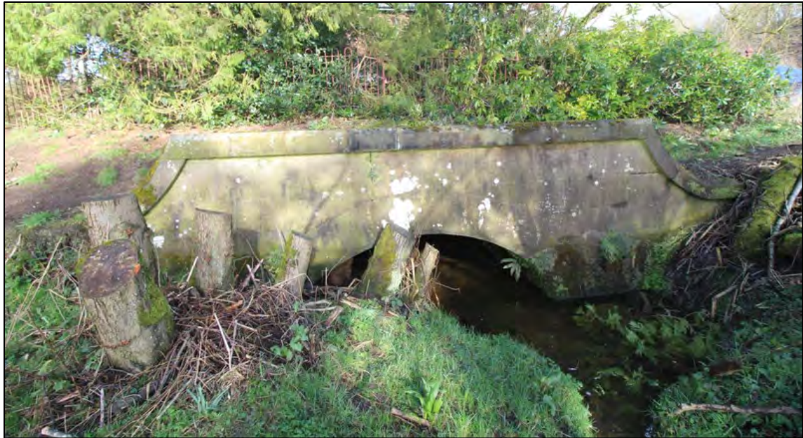
Plate 7: Ashlar opening of tail race, with overgrown boundary fence to the rear
