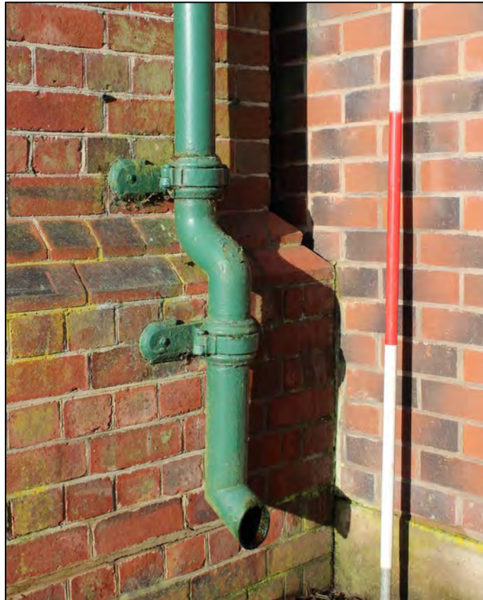
Plate 12: Detail of chamfered plinth, and cast-iron down pipe and attachment brackets
