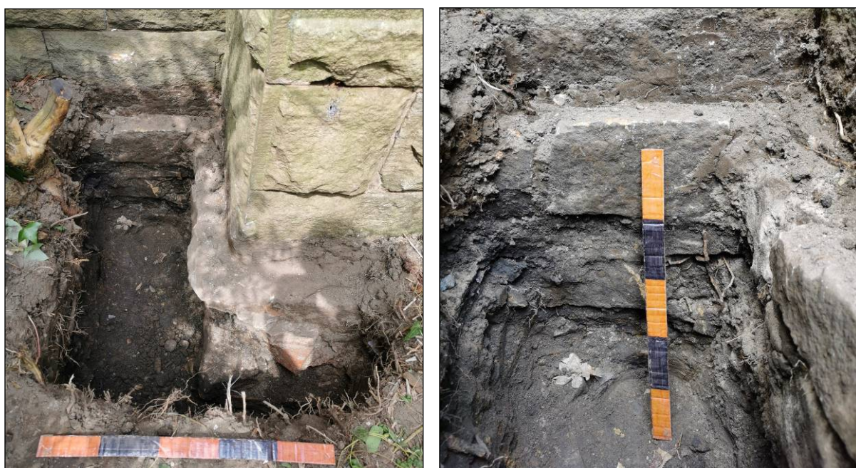
Plates 6 and 7: View of Trial Pit 1 showing the offset in the foundation and the regular coursing of the church wall, looking north
