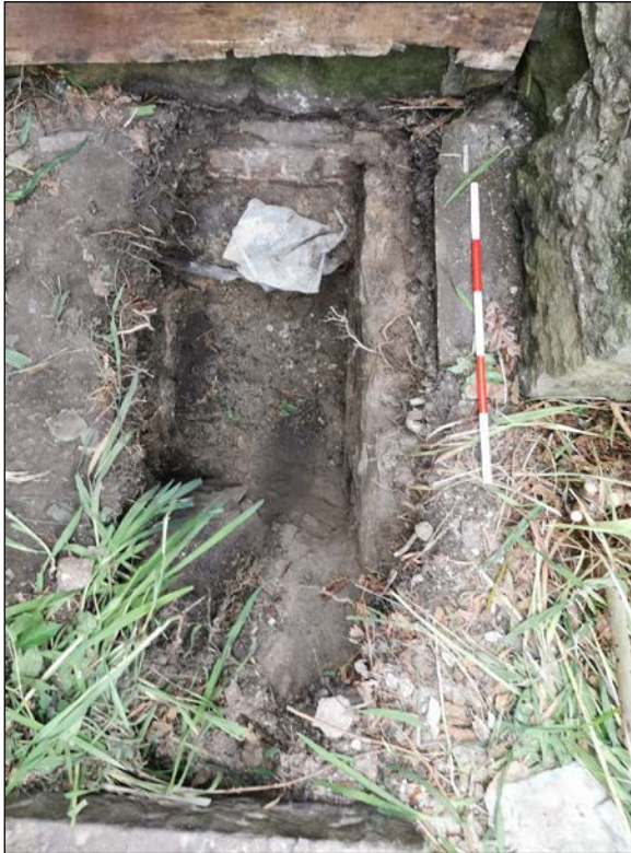
Plates 13 and 14: View of Trial Pit 4, showing wrapped concrete
