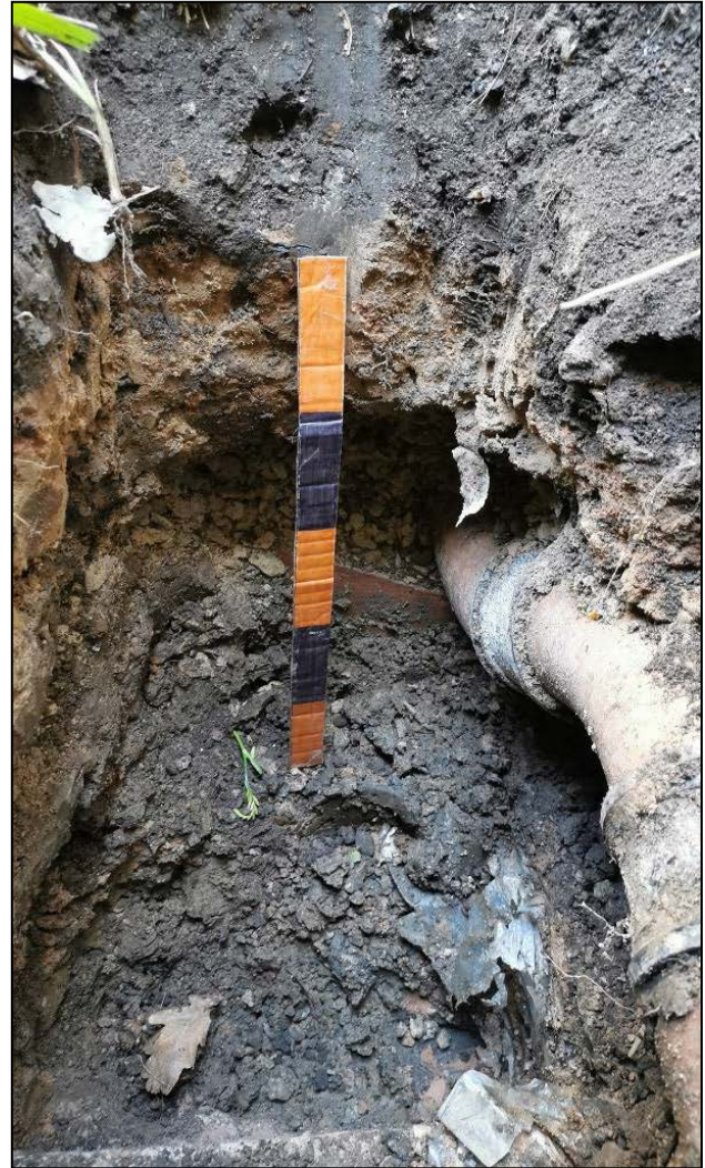
Plates 11 and 12: View of Trial Pit 3, showing the concrete raft for the 1984 extension and the surface water drain
