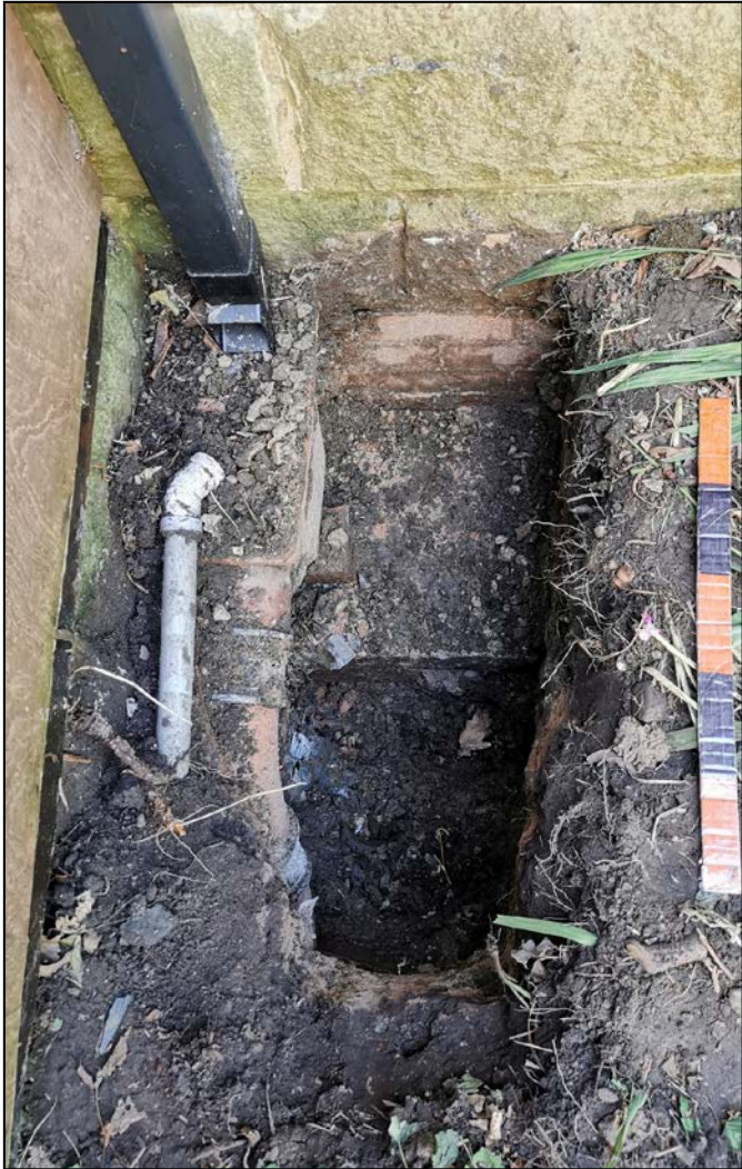
Plates 11 and 12: View of Trial Pit 3, showing the concrete raft for the 1984 extension and the surface water drain
