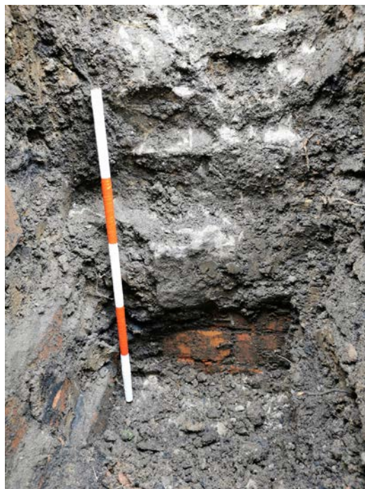
Plate 15: View of Trial Pit 5, showing brick courses below stone foundations
