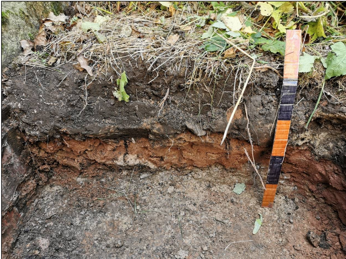
Plate 10: View of north-facing section of Trial Pit 2, looking south, showing the concrete raft and sand layer overlaid with garden soil.
