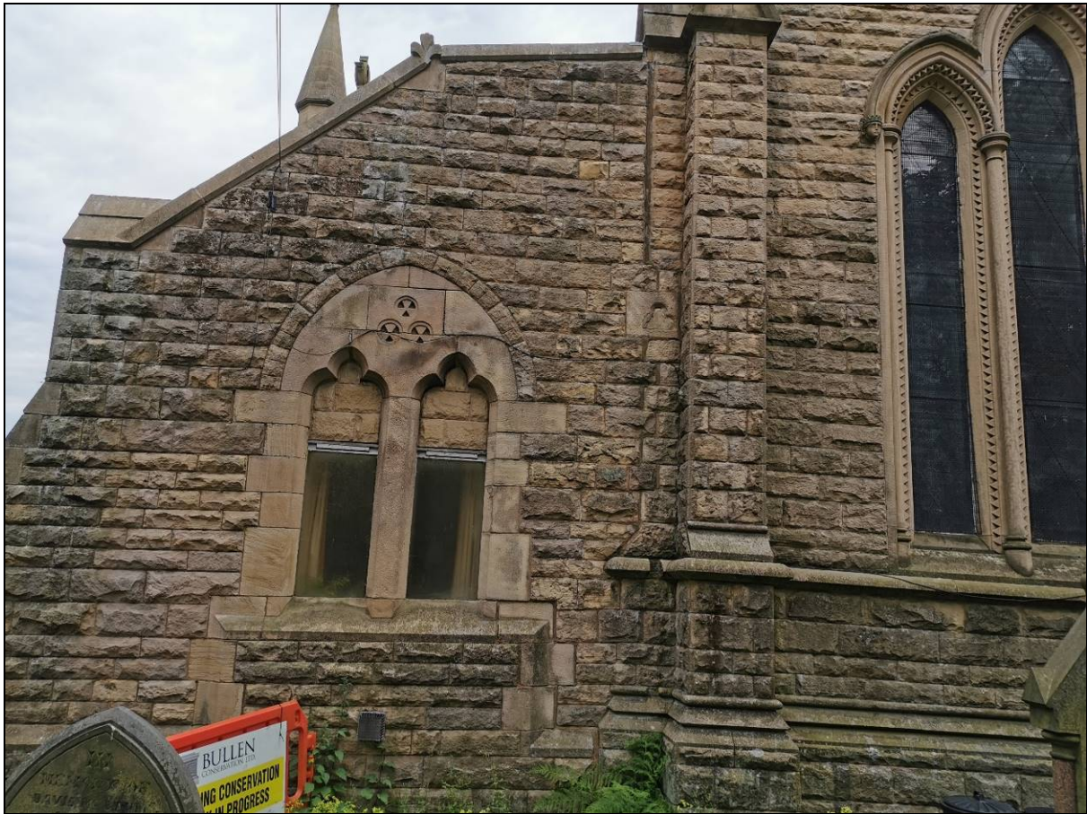
Plate 15: View of east wall showing the joint in the stonework between two phases of construction
