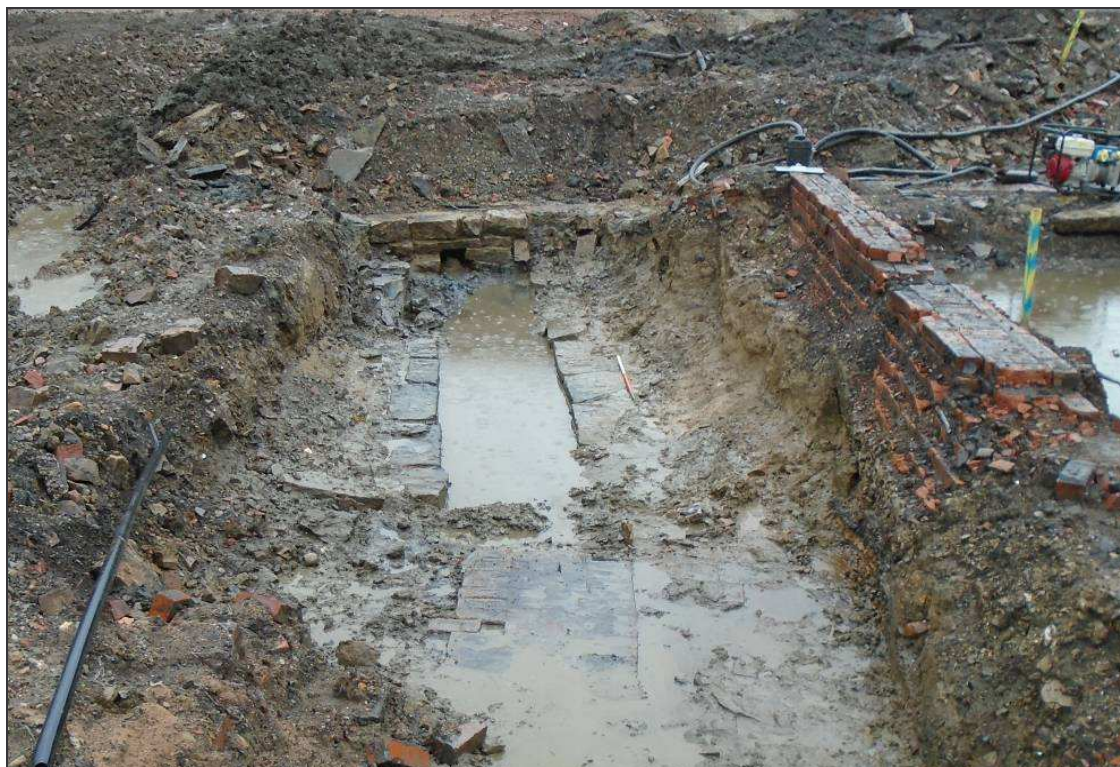
Plate 11: The truncated foundations of the waterwheel pit that had powered Salt Pye Mill, showing the brick-built wall of the twentieth-century weigh house
