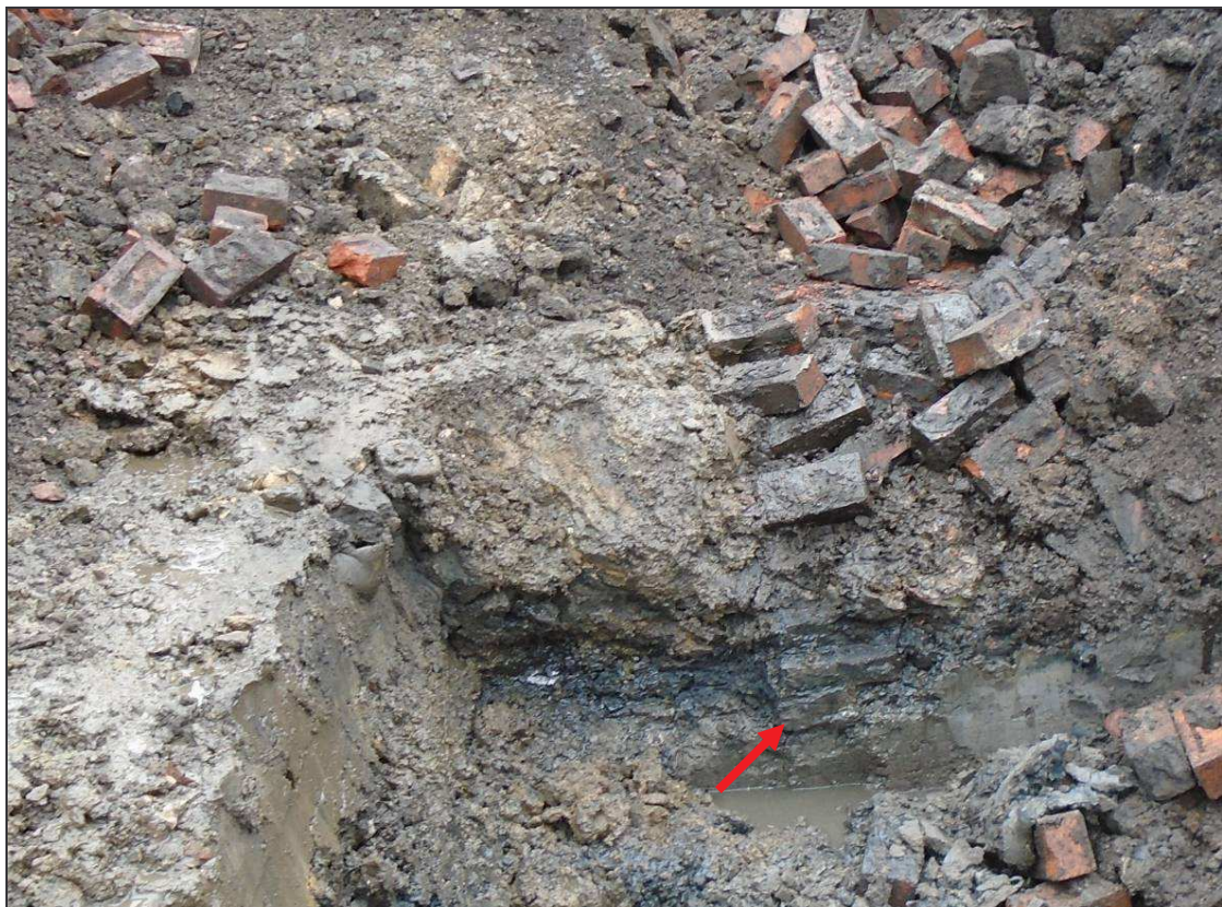
Plate 14: Fragmentary remains of the stone-built tail race, comprising a stone-built side wall (marked by the arrow) and a flat stone capping
