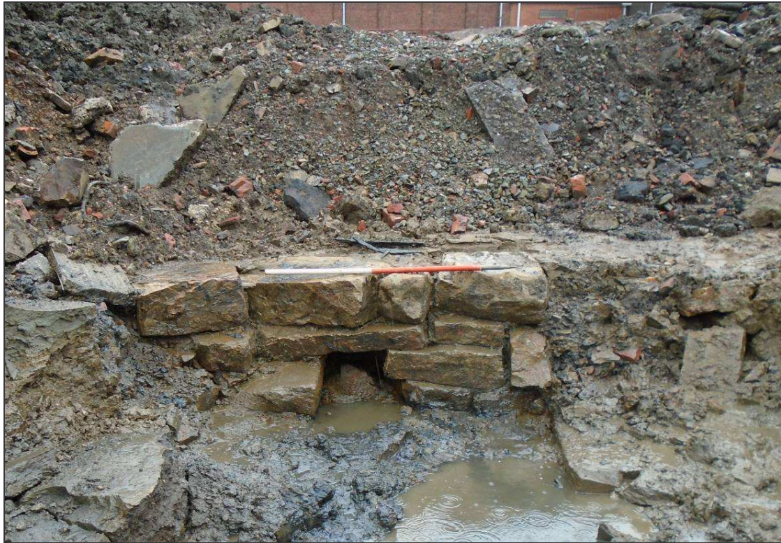
Plate 13: The stone-built north-eastern wall of the wheel pit
