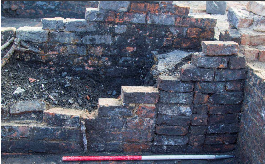
Plate 22: House B, staircase wall and bricked-up section, looking east
