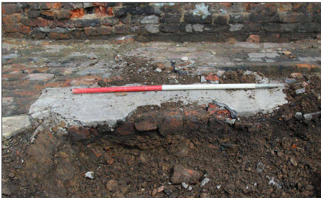
Plate 29: Sondage through the floor of House 1 showing bricks beneath the strip of concrete and natural deposits below
