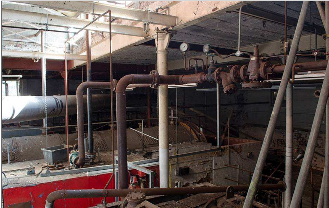
Plate 9: A view of the interior of the boiler house in 2014, showing one of the original boilers converted for use to store heating fuel (reproduced from www.28dayslater.co.uk )
