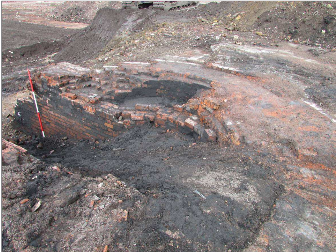
Plate 33: Inner chimney flue wall and structural brickwork to central eye. Looking north- west
