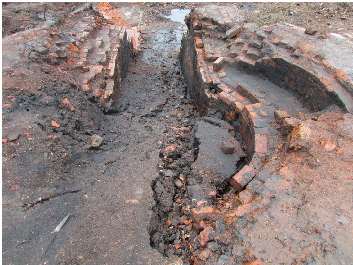
Plate 34: Exposed cross-section of the chimney stack. Looking west
