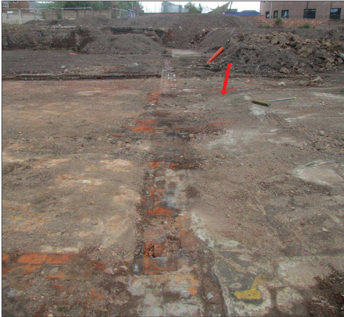
Plate 23: Western wall of the engine and boiler houses. The rope race (arrowed) can be just seen to the right
