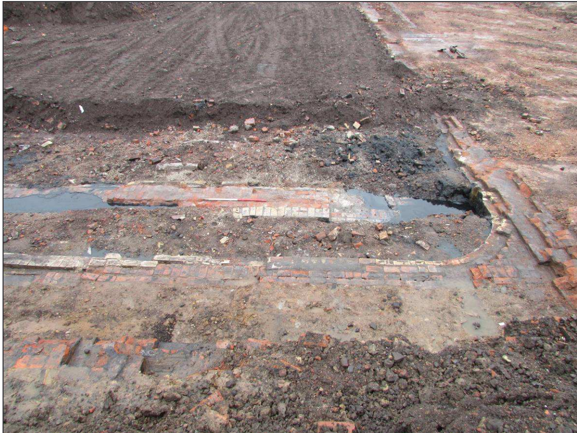
Plate 31: Elevated view of the backfilled economiser flue channels. Looking west
