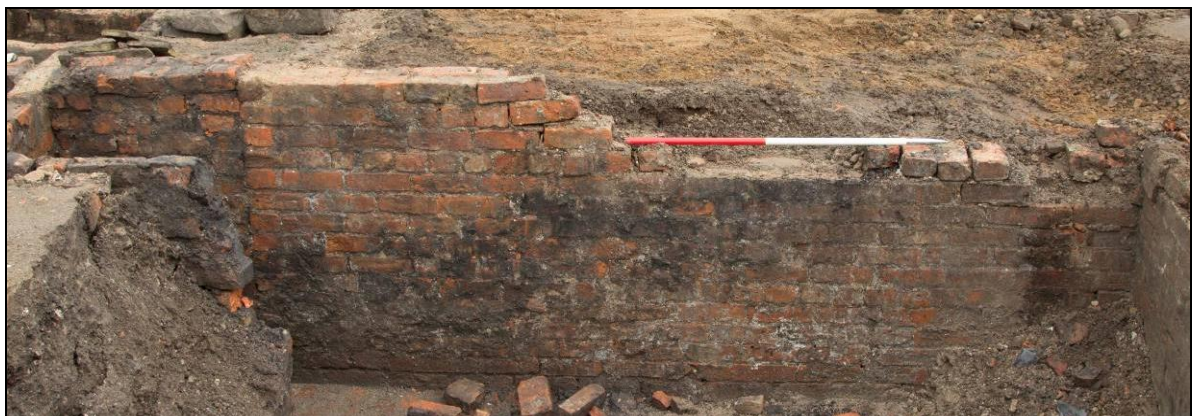
Plate 25: The northern wall of Cellar 2 showing the bricked-up doorway on the left of the photo, the wall was lowered by machine on the right of the photo to allow safe access into the cellar, looking north
