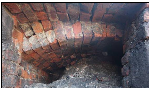
Plate 16: Detail of vaulted roof of storeroom abutting the front entrance of House B
