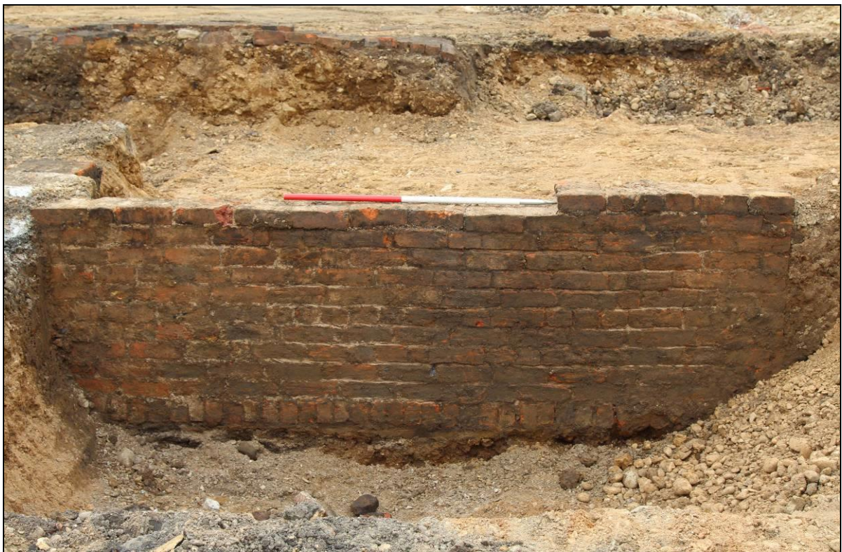
Plate 42: Early 19 th -century hand-made brick wall, looking west
