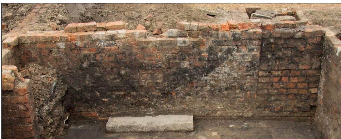
Plate 19: The northern wall of Cellar 1 showing bricked-up doorway on the right, looking north
