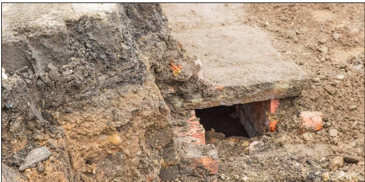
Plate 41: A cross-section of the drain/culvert at the eastern end, looking west
