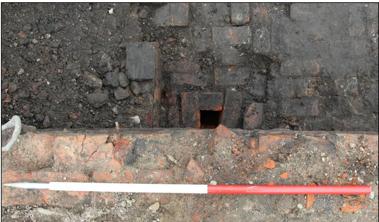
Plate 32: Brick-built drain found in the floor of Cellar 2, below the location of the stone sink
