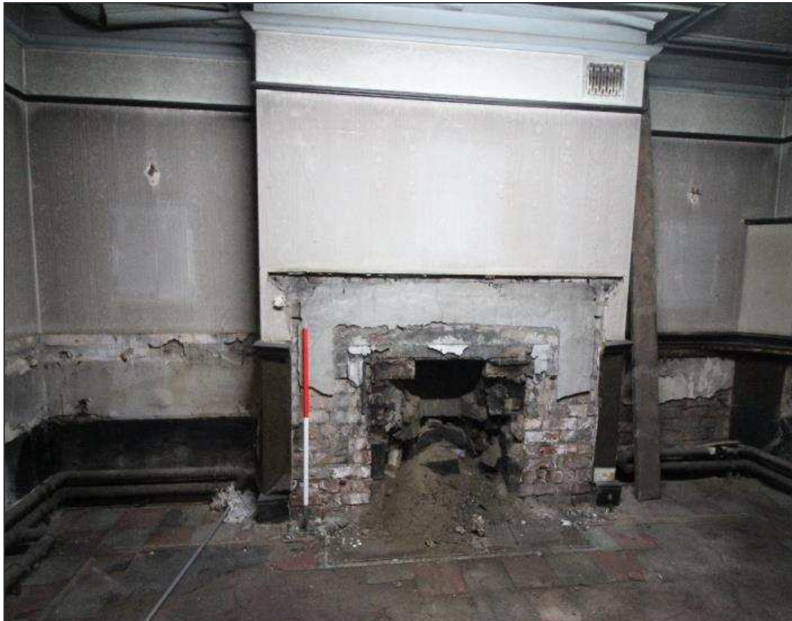
Plate 44: Protruding chimney and the robbed out fireplace in the western wall
