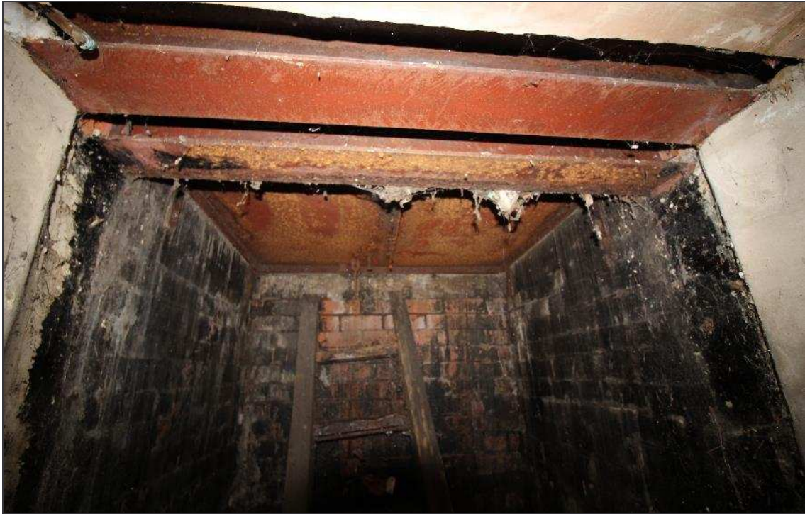
Plate 74: Cast-iron hatch doors leading to street level
