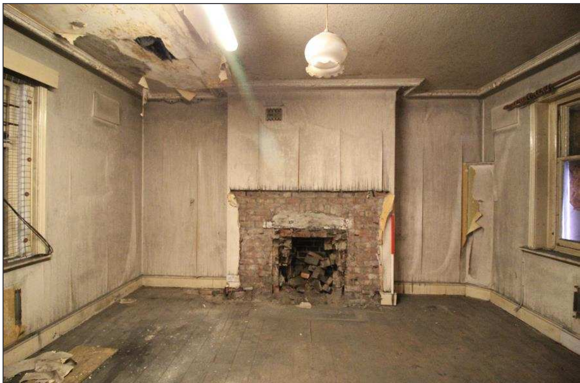
Plate 60: Chimney and robbed-out fireplace on the western elevation
