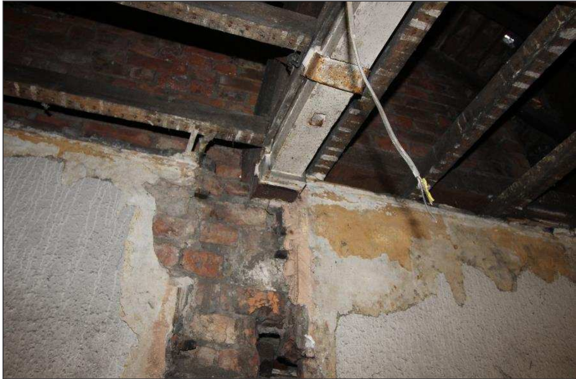
Plate 68: Detail of the tie beam support
