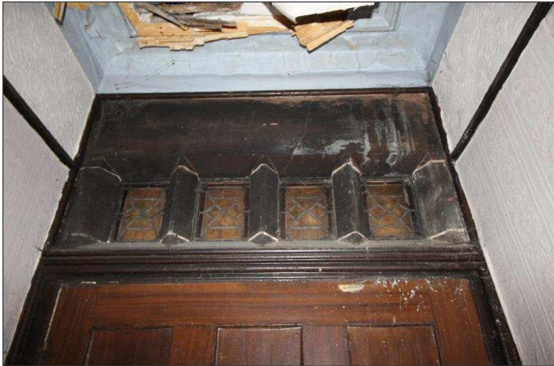
Plate 32: Detail of the sandstone mullion fanlight above the main door
