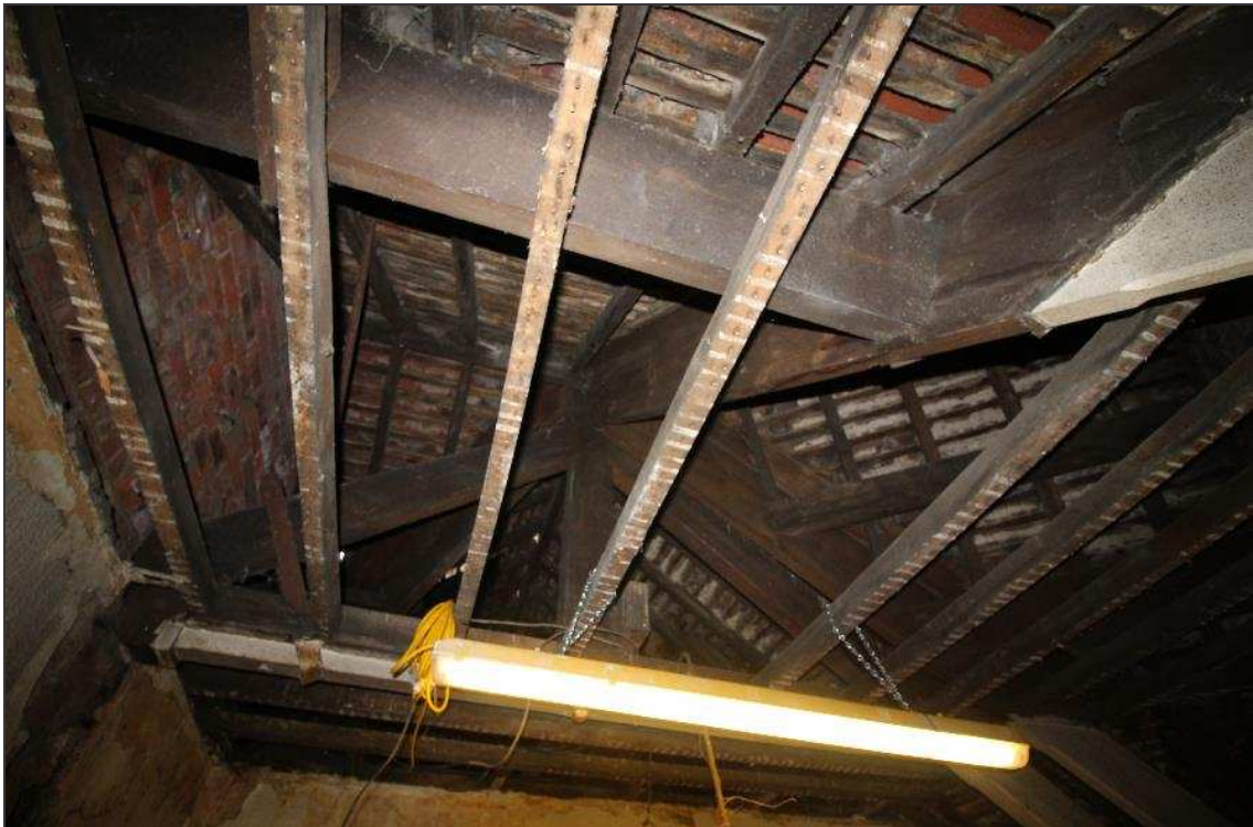
Plate 67: King post truss as seen through the ceiling joists
