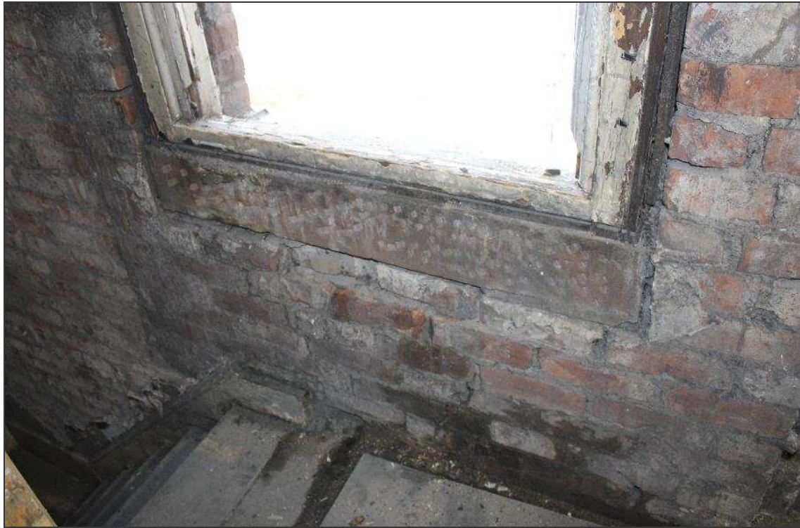
Plate 64: Detail of the original dressed sandstone sill within the western wall
