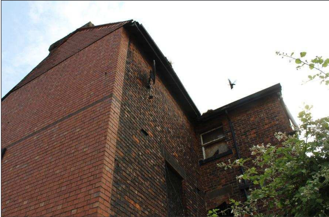
Plate 30: Detail photo of the western elevation abutting the southern elevation, denoting the rebuilding
