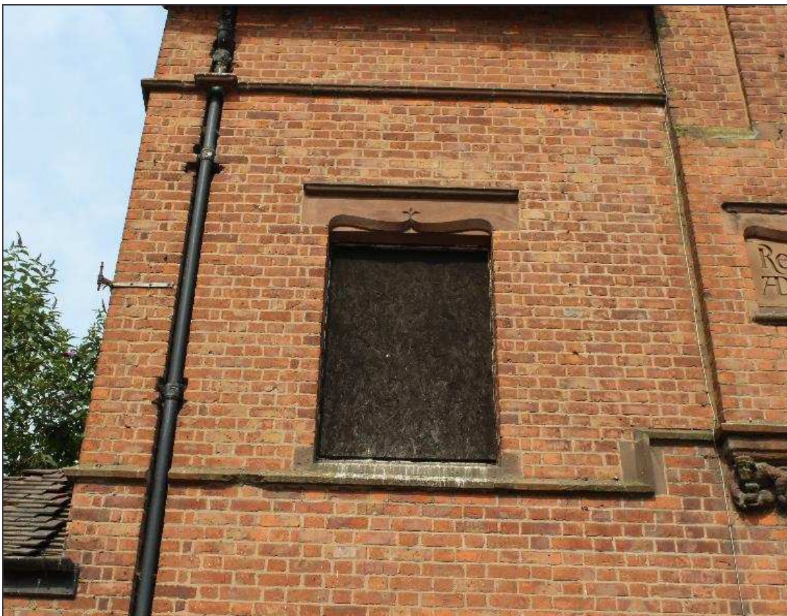
Plate 26: First-floor window detailing the swan neck carved lintel
