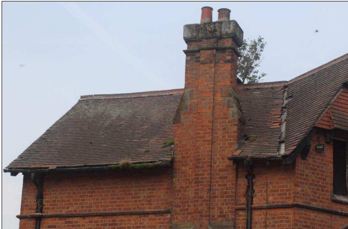
Plate 10: Detail of the slate roof along with the plain chamfered crested terracotta ridge tiles
