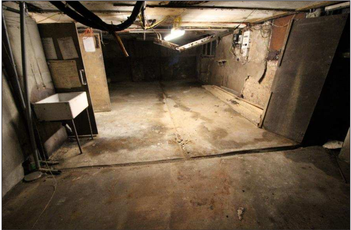
Plate 80: General view of the second room of the basement, detailing the drainage channel formed within the concrete floor
