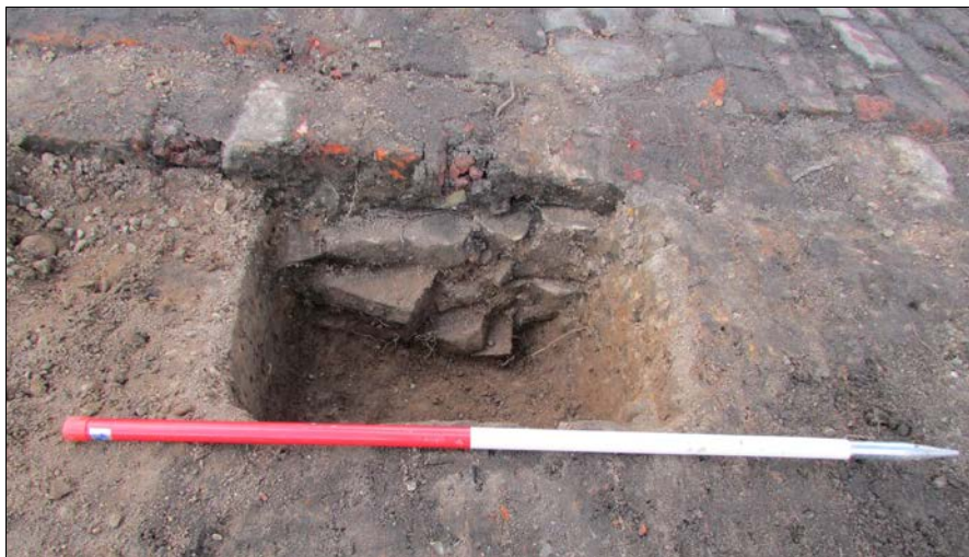
Plate 27: Stone foundations below brick wall (018)
