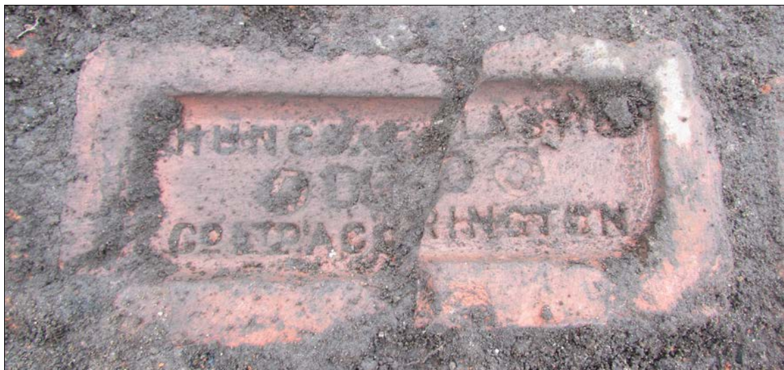
Plate 29: Frogged brick in floor surface (019)
