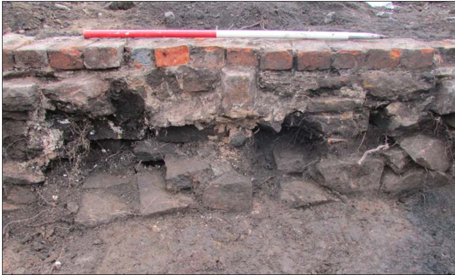
Plate 28: Stone foundations below brick wall (033)
