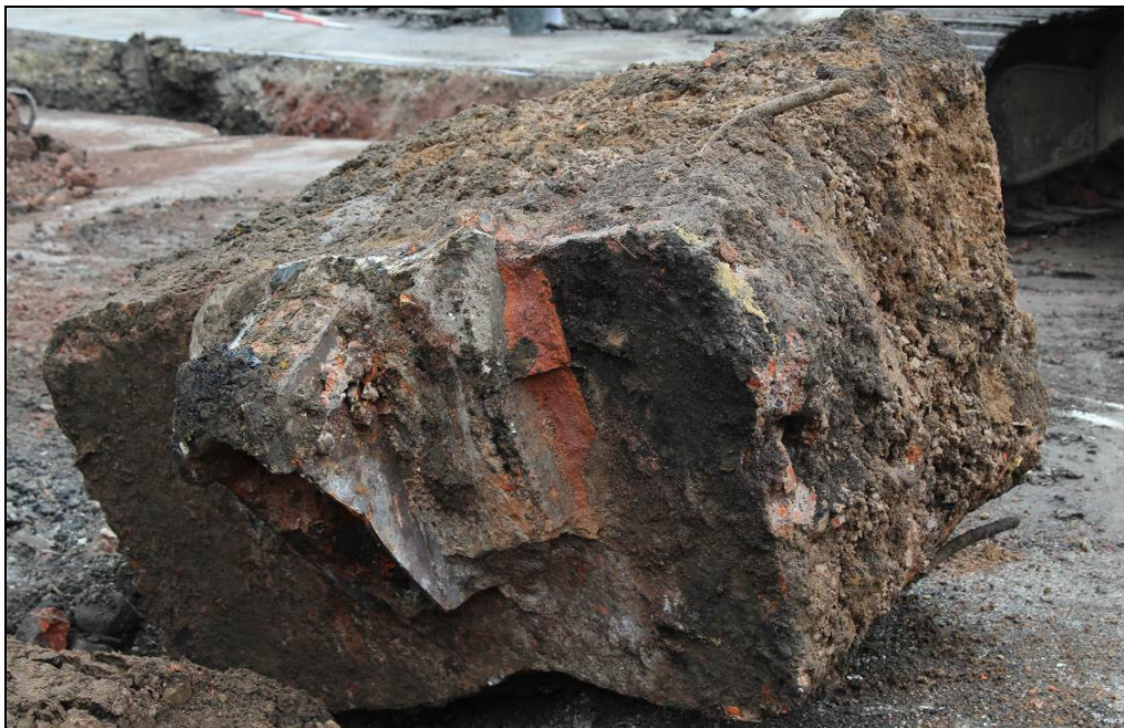
Fig. 30: A large concrete block with a cast-iron fitting on top, found next to the brick wall, suggesting this may have formed part of the main wall structure.
