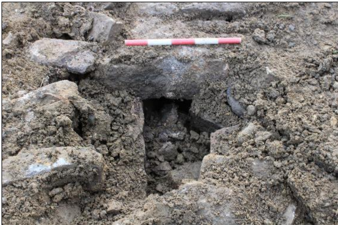
Plate 22: Close-up shot showing the interior of “French” land drain 0408
