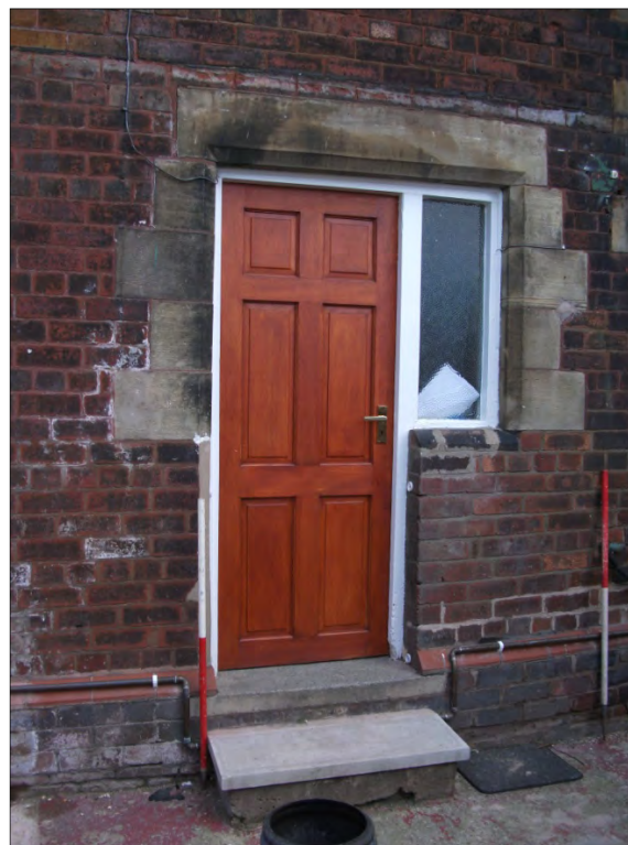
Fig 14: Former ground floor window, on south elevation which has been converted to a doorway, looking NE.
