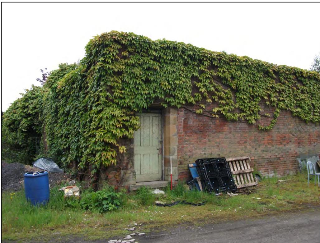
**Fig 16:** Later inserted doorway at eastern end of the gardens Northern Elevation, looking SW.
