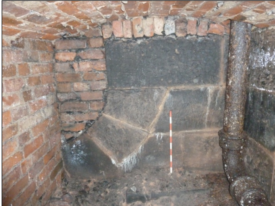
Fig 10: View of Room C4 looking at the southern wall showing a blocked stone inverted arch and heating pipe to the right.
