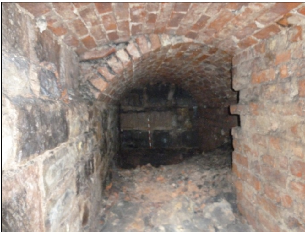
Fig 19: View of Room C12 looking southwards at the stonework beneath the brick barrel vaulting.
