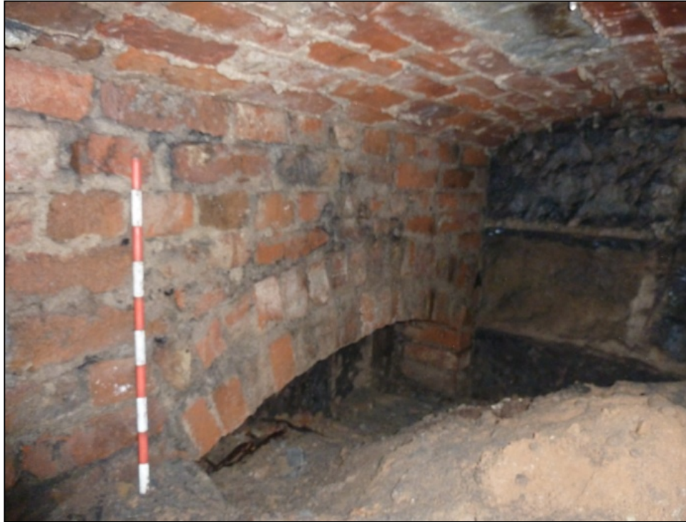
Fig 18: View of Room C11 looking south at a brick archway and what appears to be an inserted iron beam on the right.
