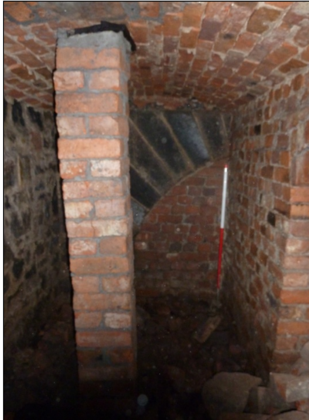
Fig 28: View of Room C26 looking north at an inserted machine-made brick pillar supporting the barrel vaulting. Note the stone arch behind.
