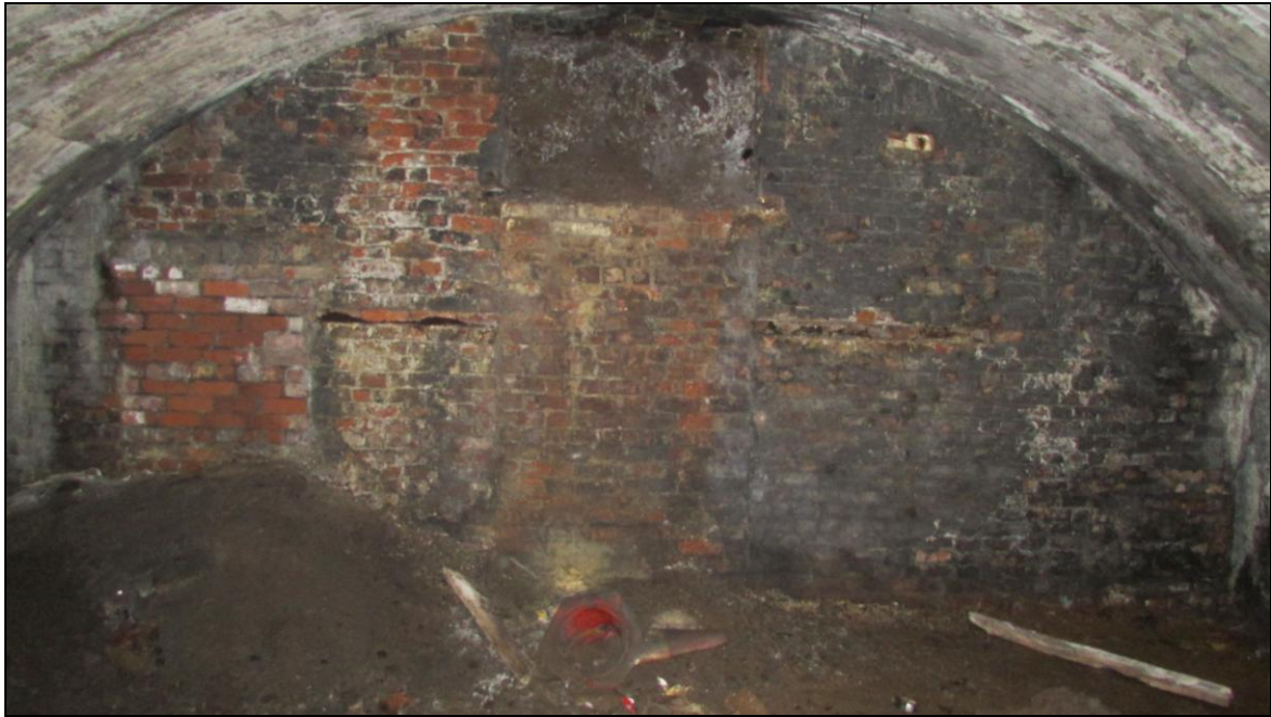
Fig. 18 The rear workshop wall, with dredged silt visible at the other side built up to the ceiling
