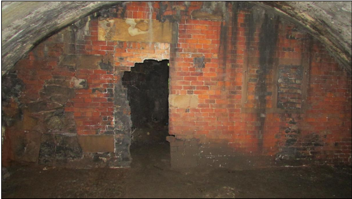
Fig. 16 Wall between the middle and rear workshop. The brick appears to have been built around the ashlar wall which can be seen on the left. Note the door and window (subsequently blocked)
