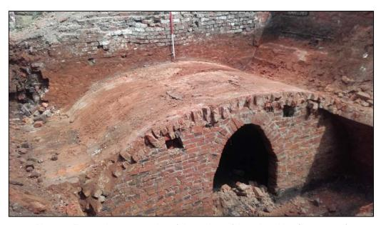
Plate 10: Exposed crown-capping of the undercroft barrel vaulting (Bay 2 open)
