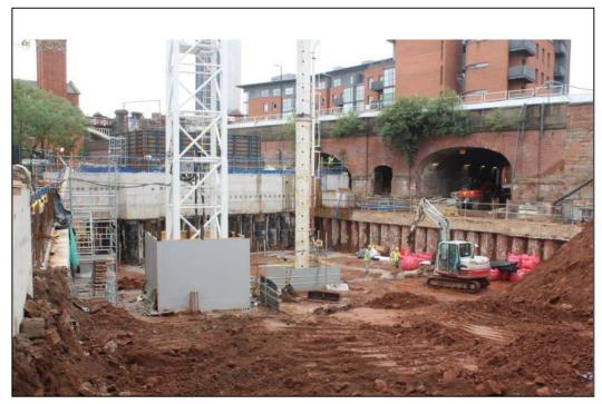
Plate 28: General view across the site during the watching brief in June 2019, showing the piling wall in place
