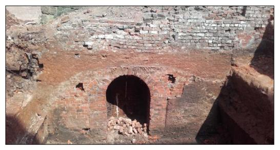
Plate 11: West-facing elevation of wall 019 showing the alcove
