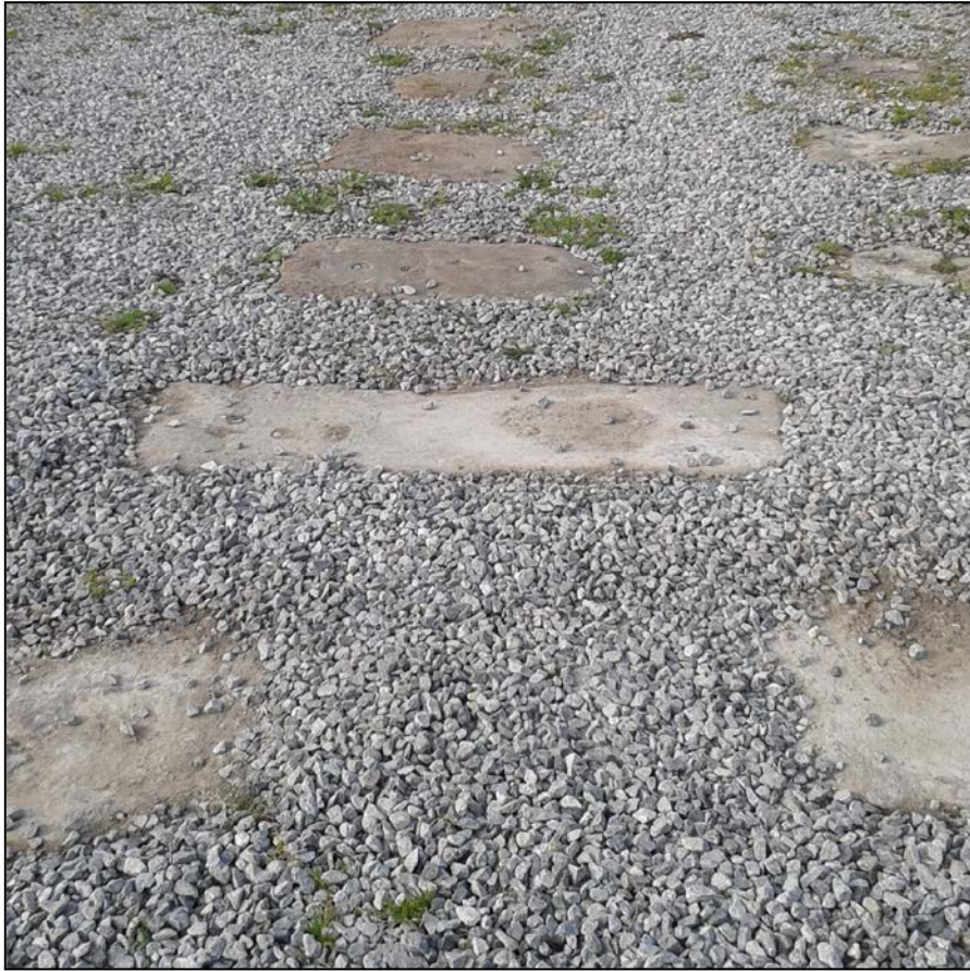
Figure 17. Examples of in situ tramway sleepers at Bugsworth Basin.
