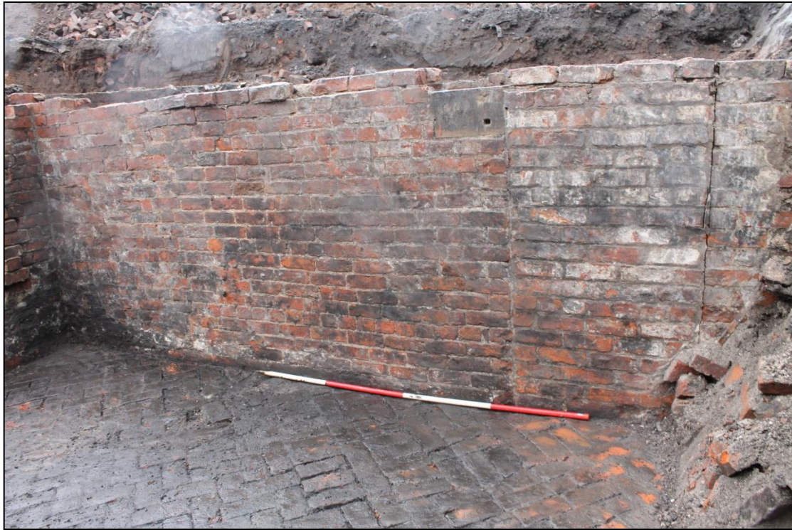
Plate 69: Wall 122, showing blocked doorway and door jamb
