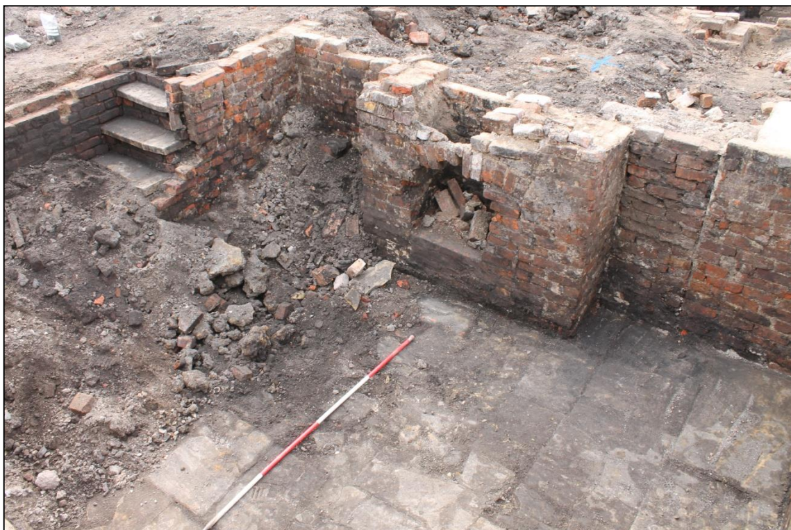
Plate 92: House 3 showing wall 172, staircase 173 wall 174 with chimney breast built in it and stone flags 175
