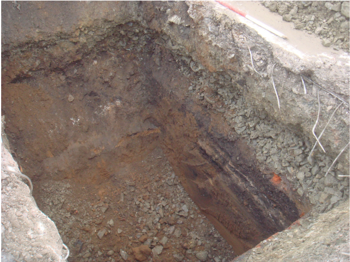
Depth of levelling material in trench 1a, natural sand at base, looking north
