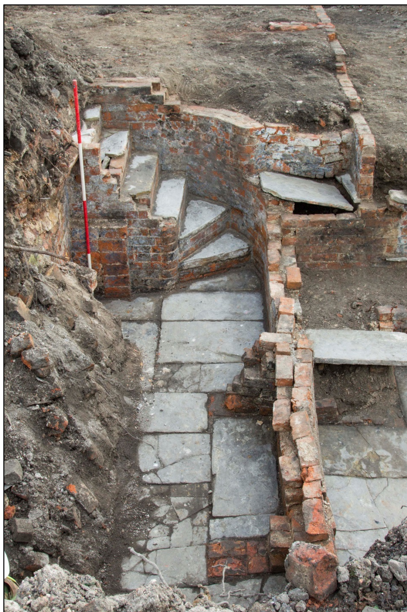
Plate 41: Staircase, flagged-floor and fireplace foundations in house 6. Springing point for a barrel vaulted ceiling visible at the left of the scale, looking south
