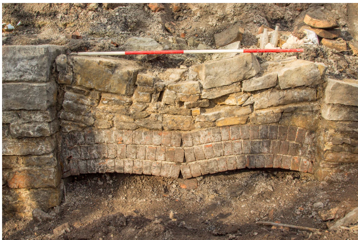
Plate 59: Slumped brick arch in the wall furthest north of the trench, looking north
