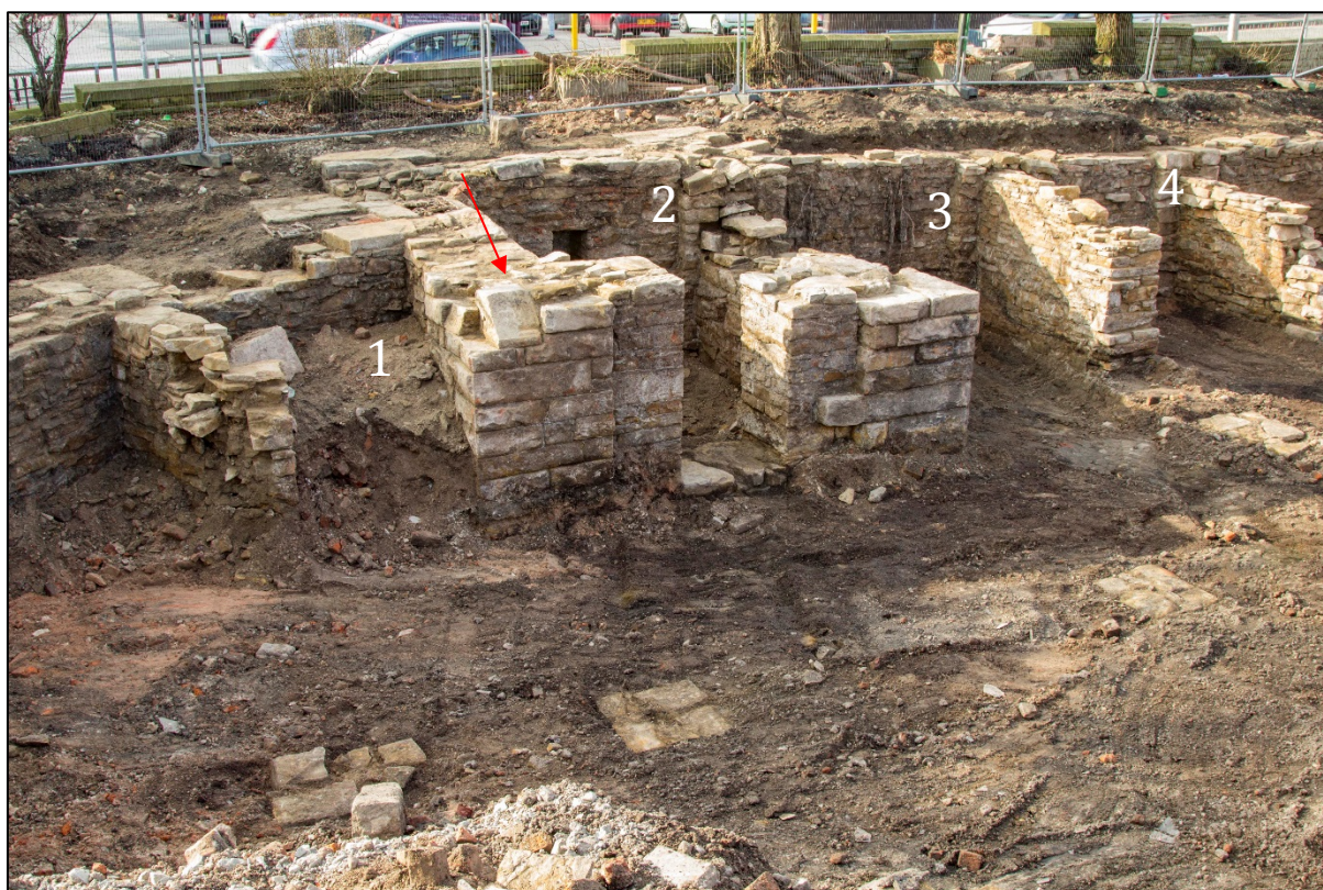
Plate 49: The western wall showing the first four bays from south to north. The red arrow shows a chamfered block indicating vaulting, looking west
