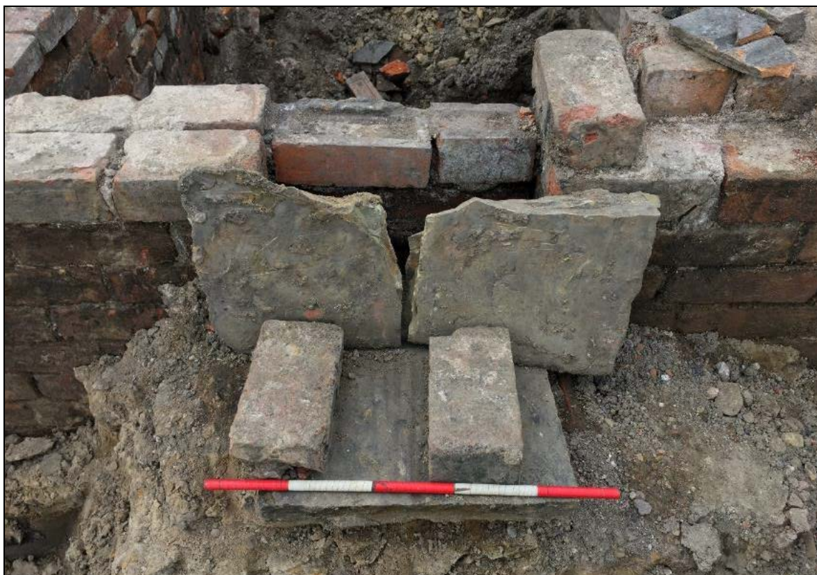
Plate 8: Blocked-up cellar light/coal chute in Room 1, looking north-west. Scale 0.50m
